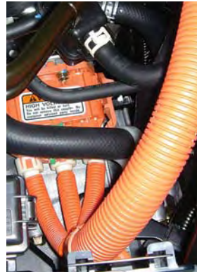
High-Voltage Cable Connection to Motor
