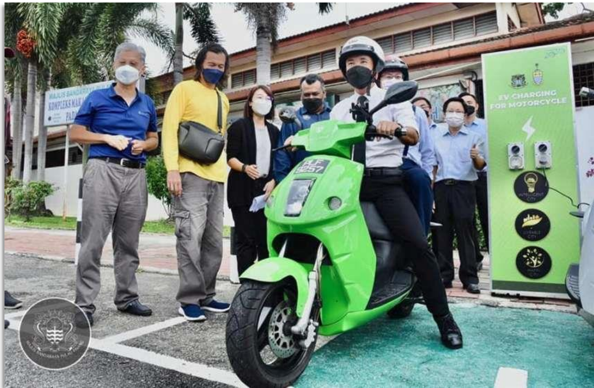
Photo 2: Electric Motorcycle Charging Station in Penang
