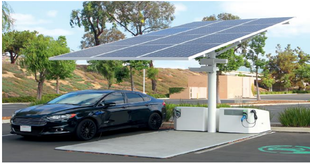
Solar Roof Panels
