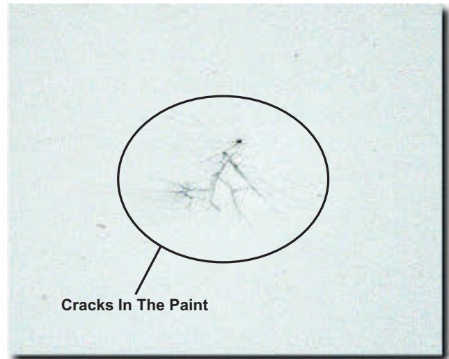
A-3 These cracks in the finish are from prying with a pick.
