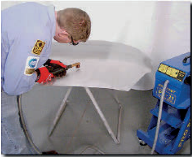
C-8 An induction heater can be used to heat a damaged area on this aluminum hood.
